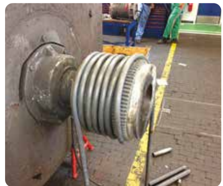
Heating a coupling for dismounting
